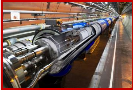
Circular particle accelerators magnet :
